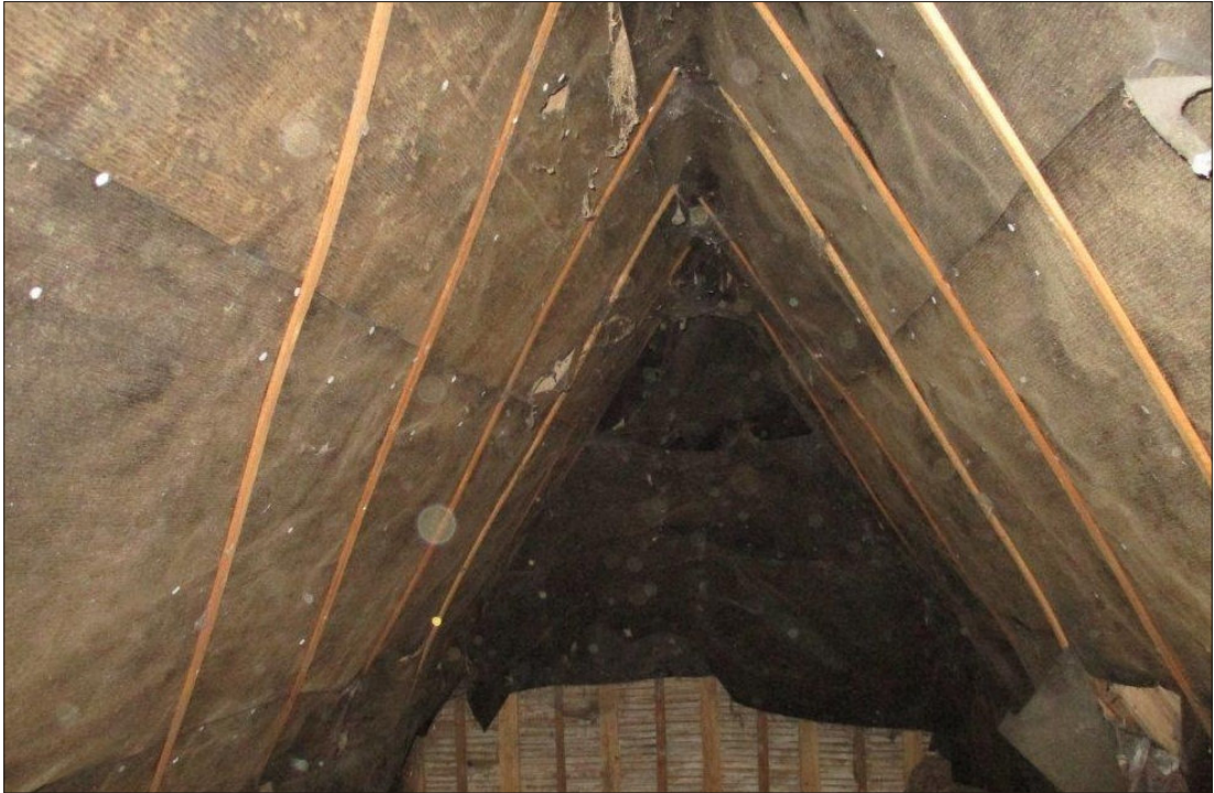
PHOTOGRAPH 13: Loft 2 of Building B7
