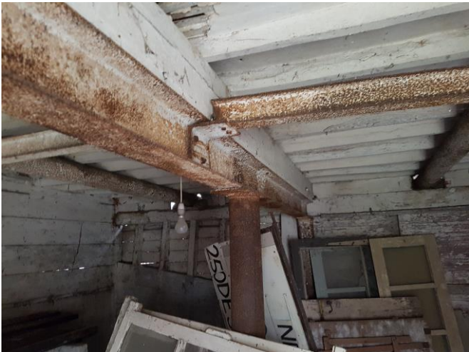
Unit 2 – Floor Strengthening
