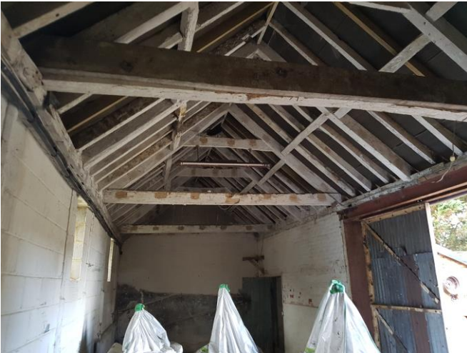
Unit 1 – Roof Structure
