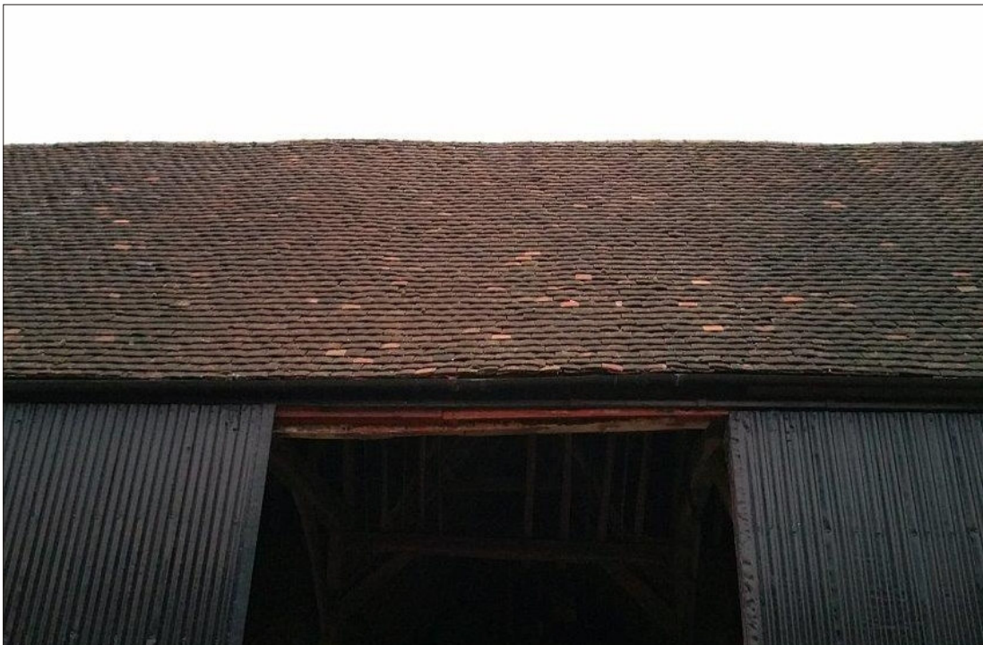
PHOTOGRAPH 10: Roof of Building B6
