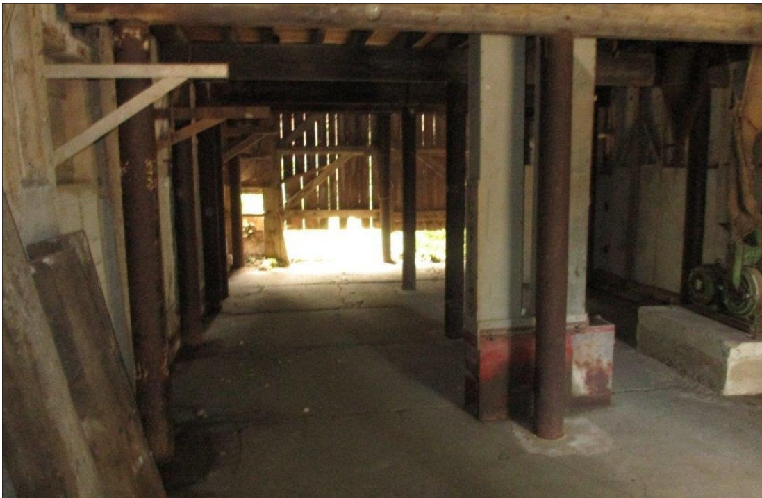
PHOTOGRAPH 6: Ground Floor Room of Building B4
