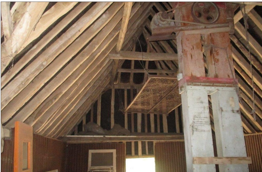
PHOTOGRAPH 8: First Floor Room of Building B4
