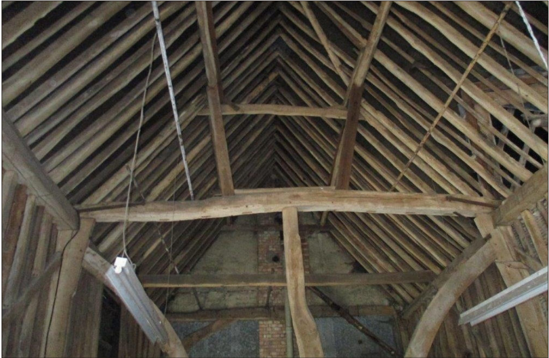
PHOTOGRAPH 11: Interior of Building B6
