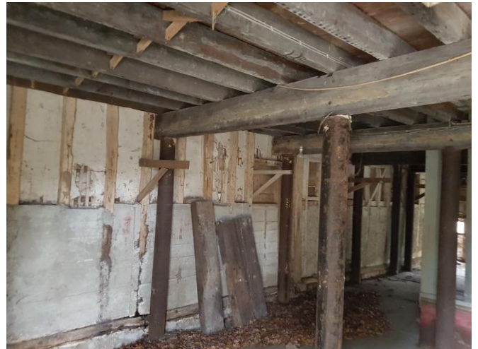
Unit 2 – Floor Strengthening
